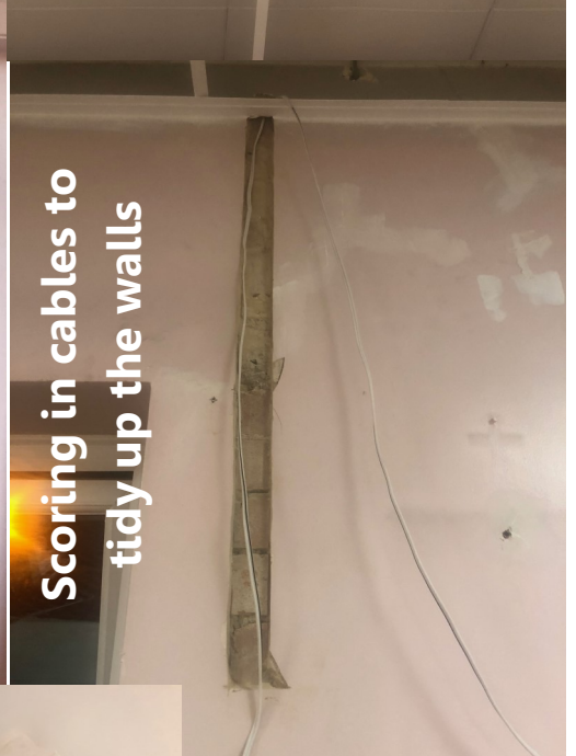
Repairing the walls
